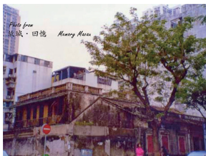
图 3 唐家花园中两层混凝土建筑 Fig.3 A two-story concrete building in Tang Garden
