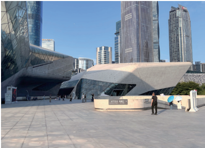
图 10 广州大剧院户外空间 Fig.10 Outdoor open space of Guangzhou Opera House
