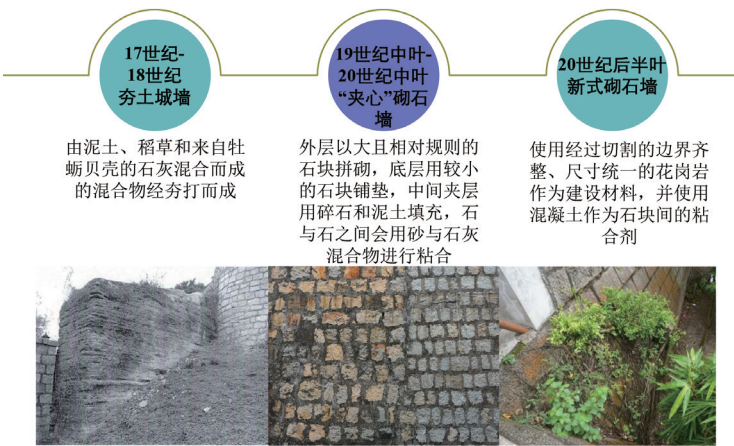
图4 澳门地区石墙砌筑工艺的发展 Fig.4 Development of stone wall masonry in Macao region
