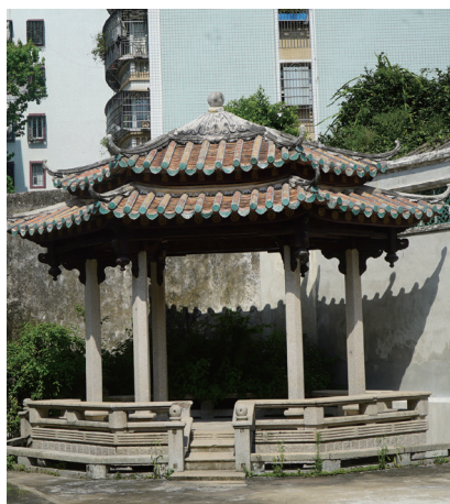
图4 西园重檐六角扁亭 Fig.4 Repeated gable hexagonal pavilion in Xi Garden
