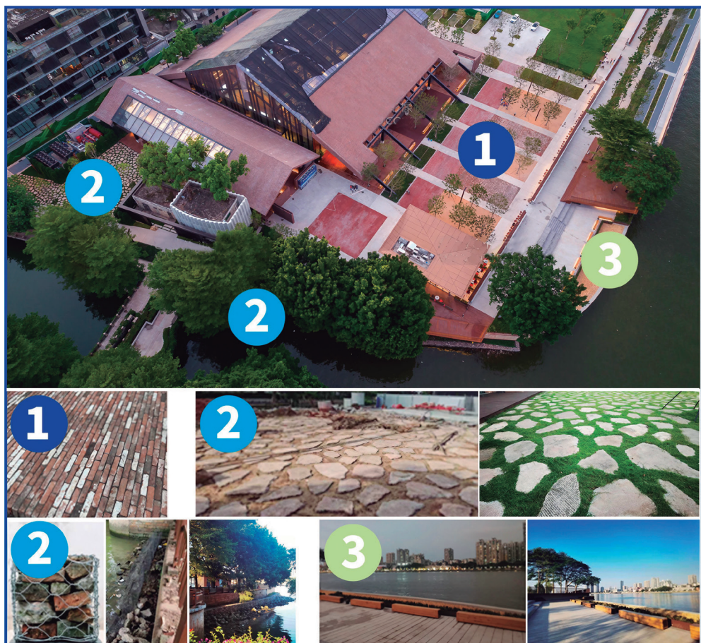
图6 红砖、混凝土、木梁的现场再利用 Fig.6 On-site reuse of red bricks, concrete and wooden beams
